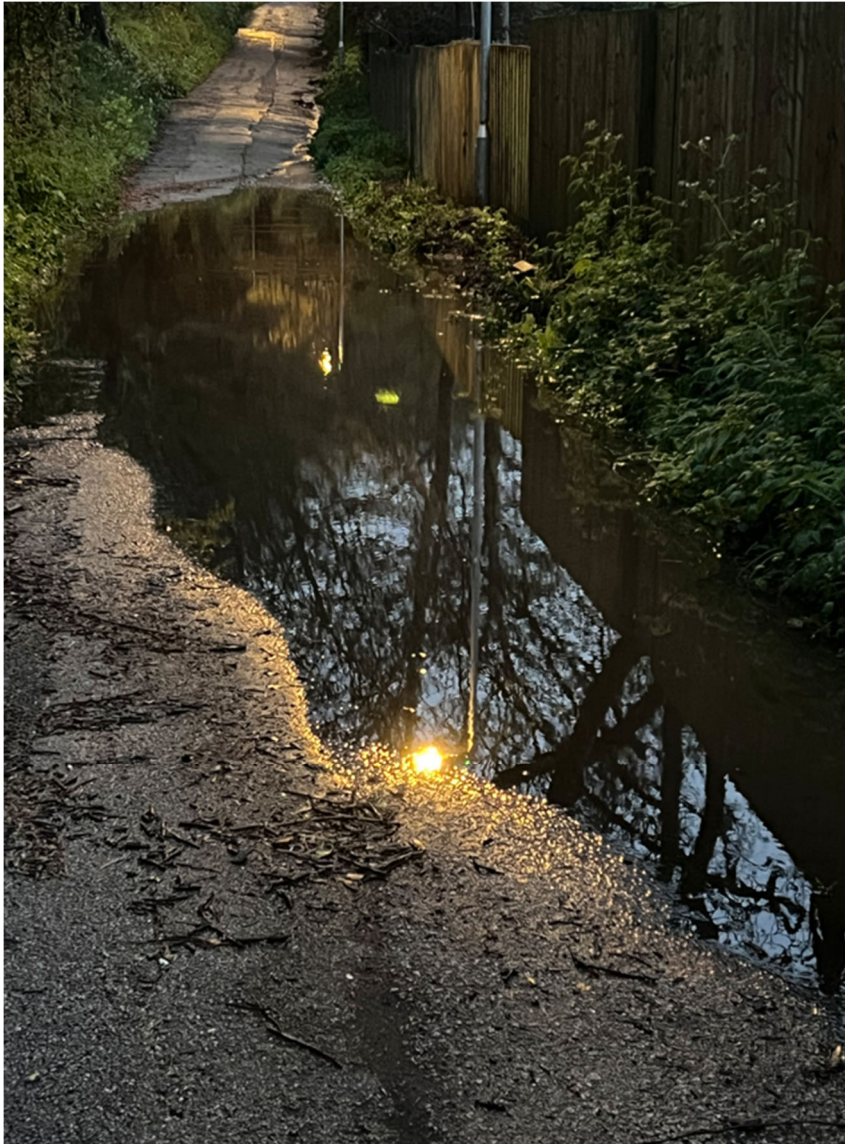
Fig 2. – surface water flooding to shared footway/cycleway from Belevedere to St Clements Hill:
